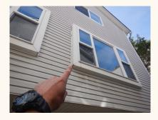
**(ED-1) Recommended Maintenance:** Localized caulking missing/failure was noted on the exterior - see siding and trim junctures and window frames and in some trim. Preventative caulking maintenance can help keep these areas weather proof and prevent water damage to materials. Have the exterior further evaluated and re-caulked and painted as needed.
