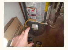
**(P-8) Repair (Minor):** The expansion tank for the water heater is corroded. This should be replaced in the near term to ensure reliable performance.
