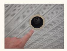
**(G1-2) Repair (Minor):** Recommend installing a cover for this light bulb to prevent injury or electrical issues related to damage. Location under stairs in garage as well as ceiling.
