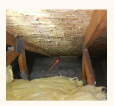
(A-2) Efficiency: The attic insulation could be improved to modern standards, which recommend R-49 on the floor and R-21 on walls. During insulation repairs it is best practices to implement any air seal-up repairs to seal air leakage.
