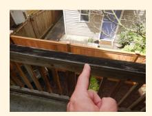
**(ED-7) Repair (Moderate):** The deck handrail and guardrail is loose and may not be adequately prevent a falling adult. Hire a licensed general contractor to evaluate and repair / strengthen this deck guardrail system to ensure safe and reliable performance.
