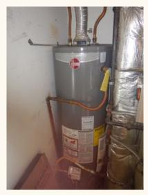
Q (P-10) Due Diligence: This water heater appears to be using F.V.I.R technology. Prior to 2003 most gas water heaters had an open combustion system which made them a potential ignition source in places like garages where gasoline vapors could ignite. Starting in 2003, residential water heaters began using "F.V.I.R." (Flammable Vapor Ignition Resistant) technology. This means that the combustion chamber is now likely sealed. Recommend confirming.
