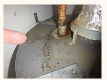
**(P-9) Repair (Minor):** The discharge tube for the water heater temperature and pressure relief valve (TPRV) is plumbed using a corrugated supply connector. Though this is very common, **this restricts the diameter of the opening** and is unsafe and not recommended - see attached link. Ideally, the discharge tube for a relief valve:
