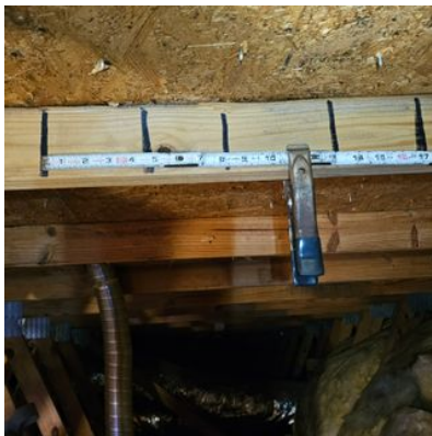
Roof Deck Attachment
