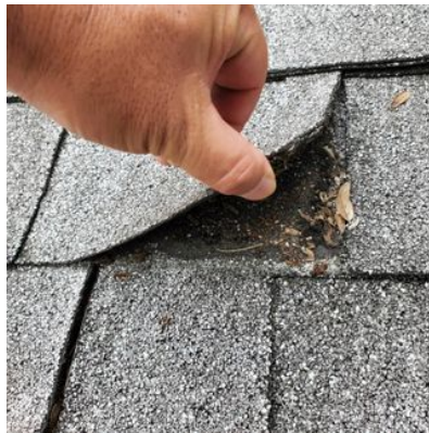
Loose shingles at multiple locations
