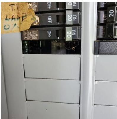
Open socket at the main panel
