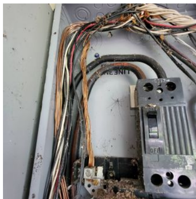
Improper grounding inside the main panel
