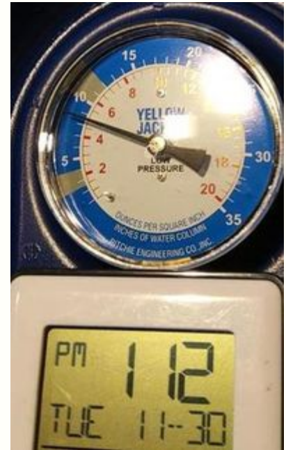
LP Leak Test - Completion
