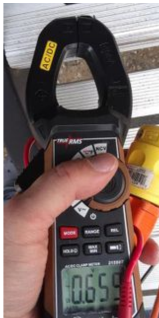
No Excessive Voltage at Steps
