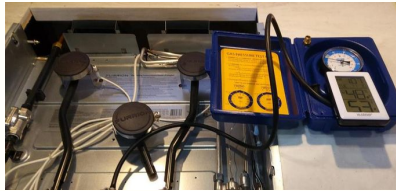
LP Leak Test Overview
