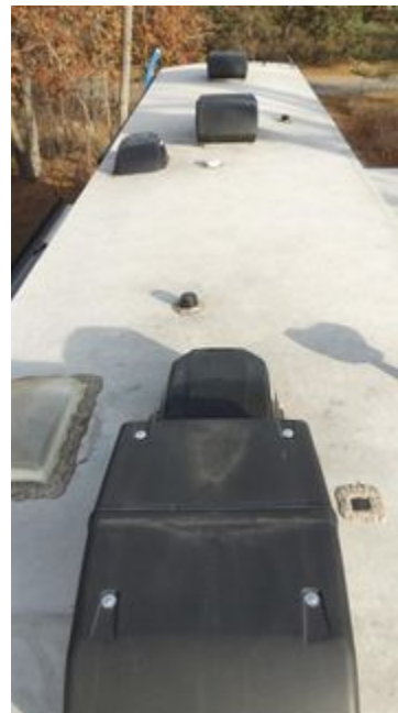
Roof Overview - Front to Back
