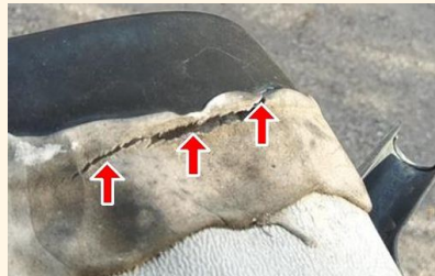
Streetside Rear Roof Sealant Gap
