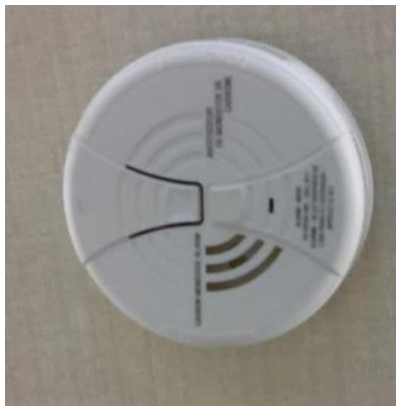
CO Detector - Front CO Detector
