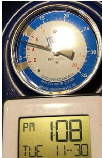
LP Leak Test - Start
