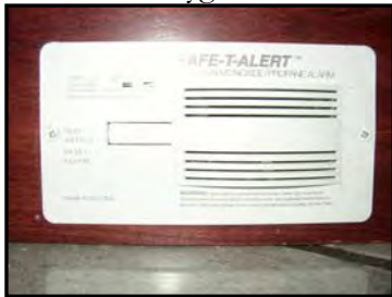
Figure 4-14. Carbon Monoxide/LP Gas Detector
