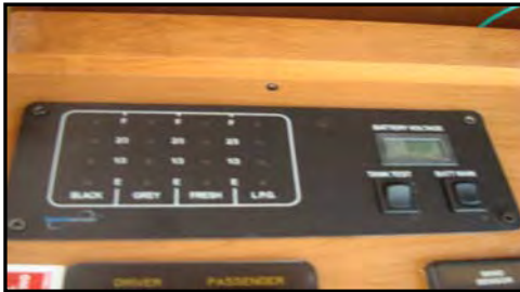
Figure 11-1. Monitor Panel (Water, LP Gas, Battery)
