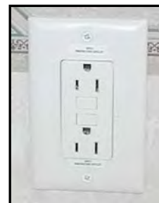
Figure 7-5. Typical AC Receptacle
