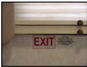
Figure 12-2. Emergency Exit Window
