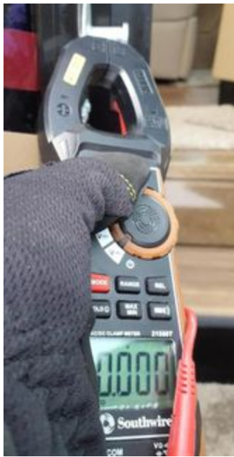
No Excessive Voltage at Entrance Door
