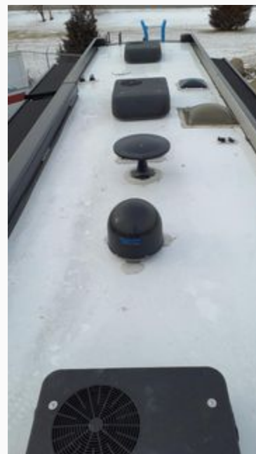
Roof Overview - Front to Back
