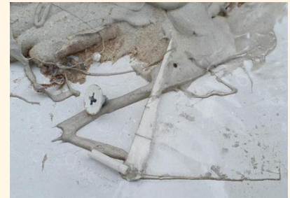
Screwhead in Sealant
