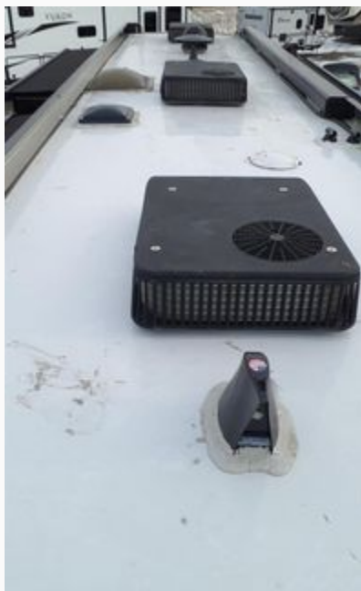
Roof Overview - Back to Front
