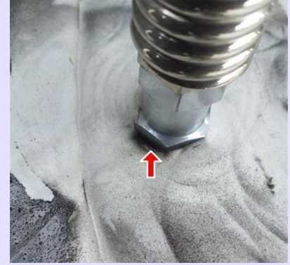
Curbside Antenna Sealant
